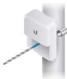
2. Drill a pilot hole into the pole.
